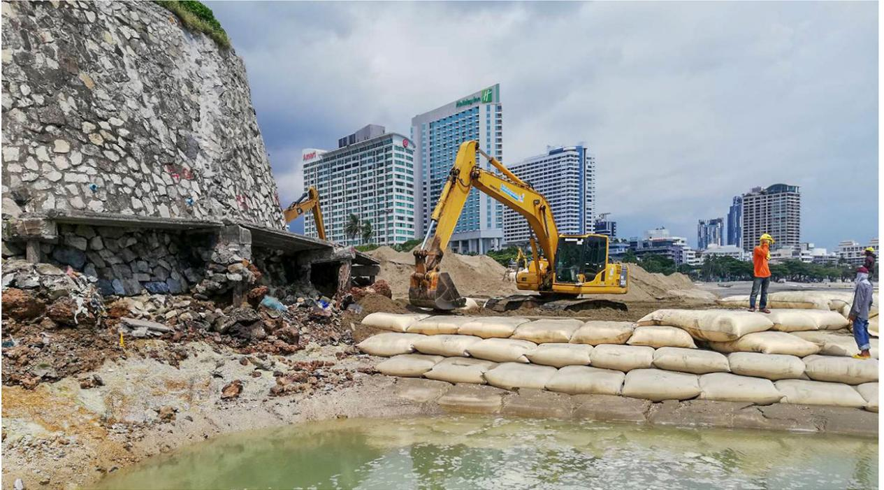
The seaside resort of Pattaya on the Gulf of Thailand, south of Bangkok, provides an exemplary case. There, geotextile sand containers (Secutex® Soft Rock RS 801a) were used as ballast and a geotextile filter (Secutex®) was installed on the subsoil near the waterline. **This revetment solution, subsequently covered by a sand protection layer, was engineered to maintain the beach surface area and enable expansion.**
