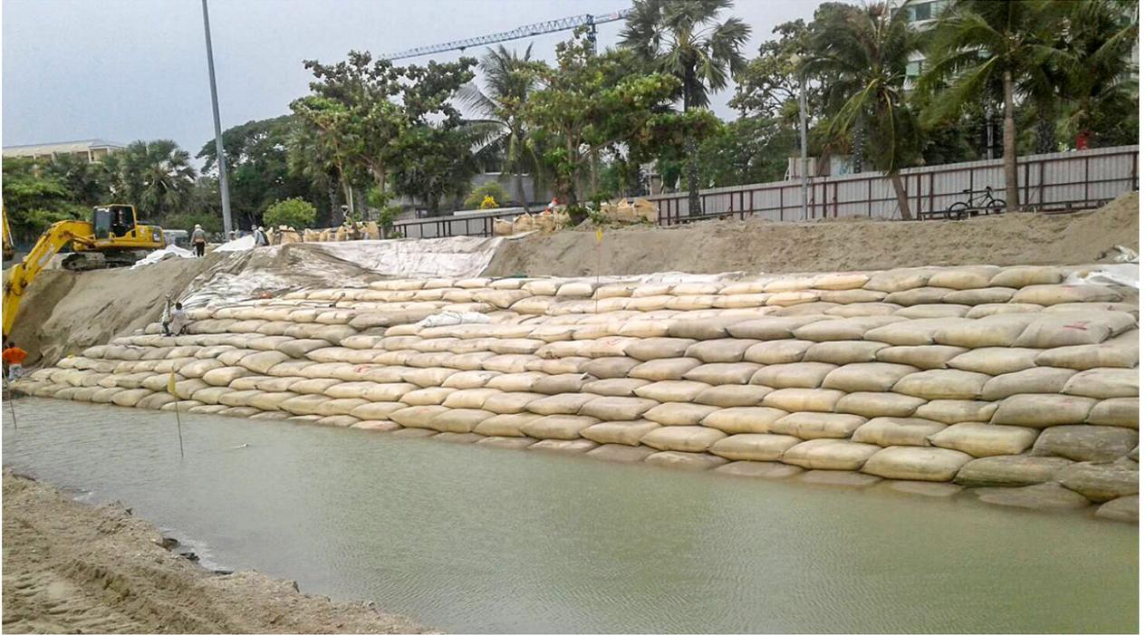
The **Secutex® Soft Rock RS 801 geotextile sandbags** and sand containers were supplied with a beige color. This enabled the 28,000 containers to blend in with the surrounding beach. Each container used a filling volume of 1m<sup>3</sup> and were filled with sand from the project site itself, which provided considerable savings for the project owners and greatly reduced material transportation needs to the site.
